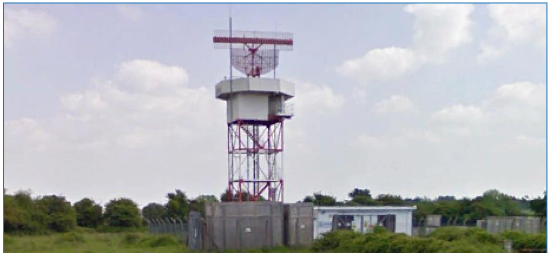
Figure 2: Shannon Airport PSR with co-mounted MSSR
